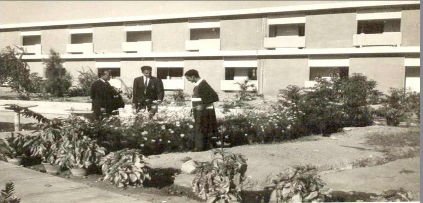
IBA Main Campus Hostel Year: 1968-69
